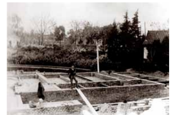
Construction of the foundations for the Barcelona Pavilion. Notice how Mies van der Rohe accepted to do the foundations out of walls made of bricks,
